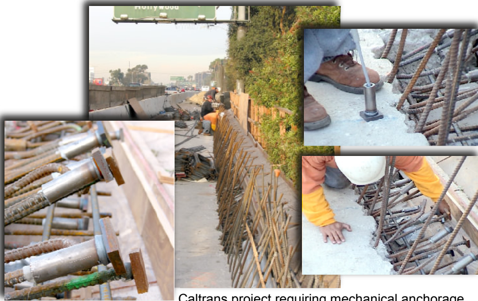
Caltrans project requiring mechanical anchorage to be installed onto existing reinforcement.
